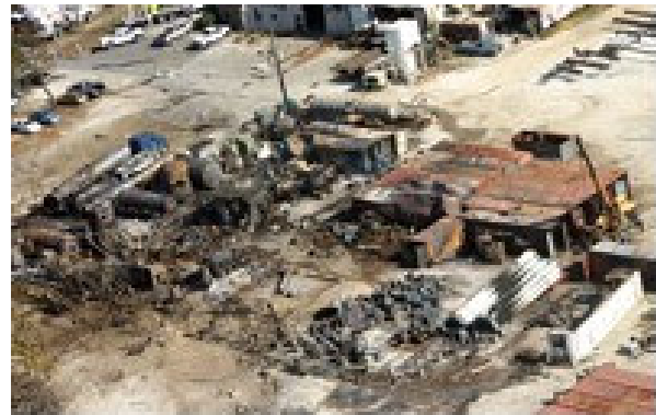
Aerial view of site after blast from CSB bulletin
